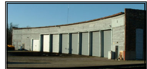
New doors installed.
