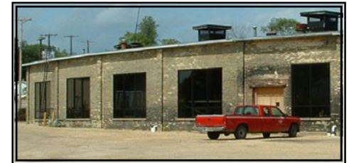
New windows installed.
